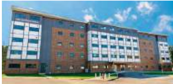
Trinity Western University’s Jacobson Hall student housing facility in Langley won Metric Modular the General Contractor Award for projects valued up to $15 million at the Vancouver Regional Construction Association Awards of Excellence last October | SUBMITTED
