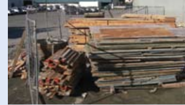
Formwork plywood and dimensional lumber stacked for recycling
